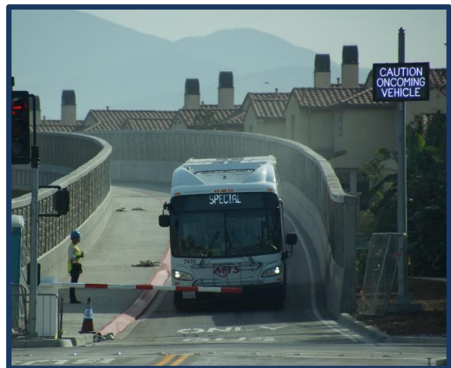
Figure 4.7 Bidirectional BRT Lane Guideway Control System, San Diego MTS (source: Arcadis IBI Group)
